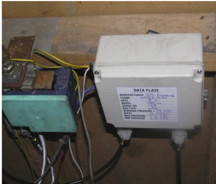
The TFLGLL Data plate is attached to the front of the Electrical control box.
